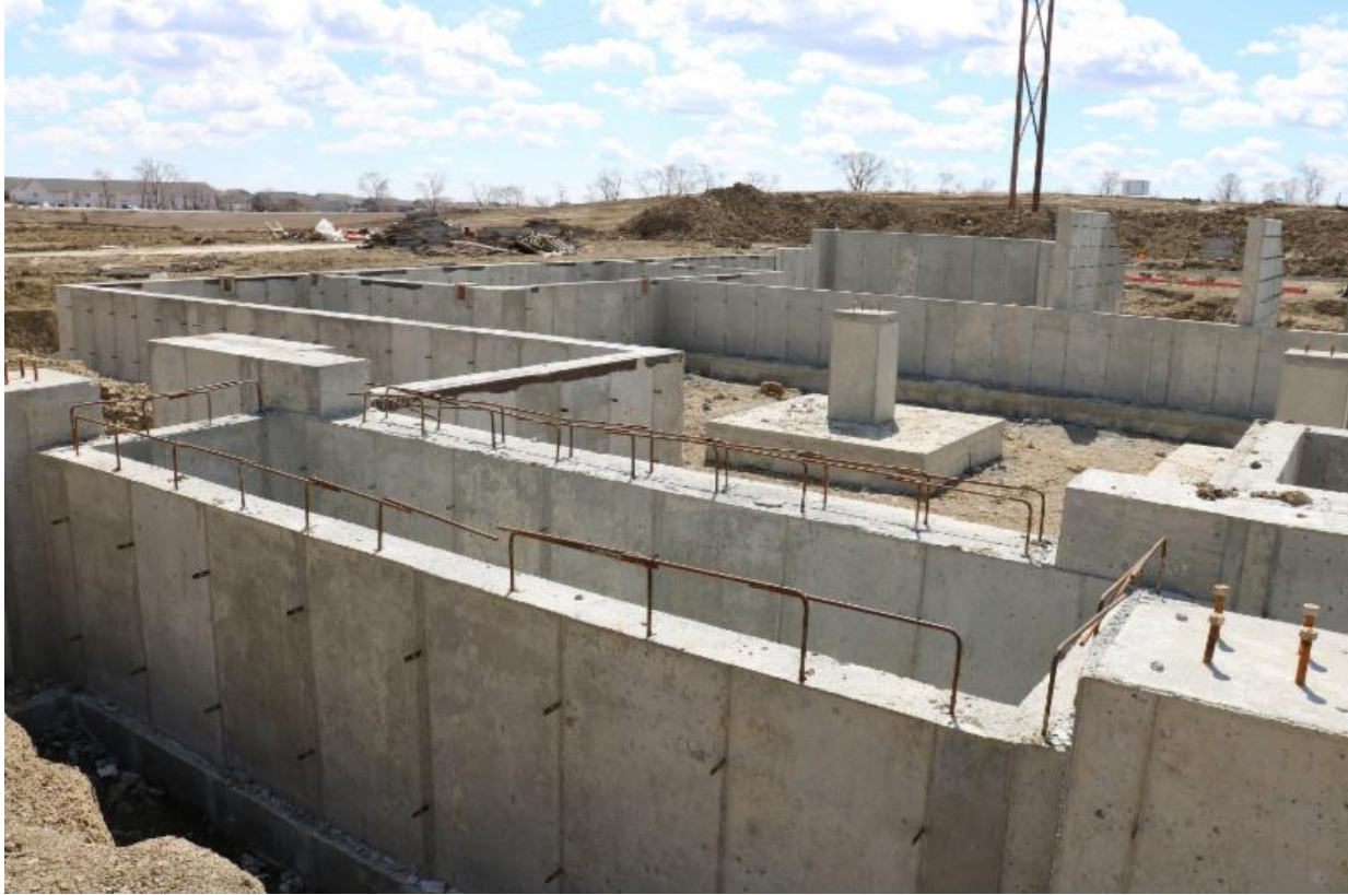
This photo shows the footings of the Fine Arts Center.
