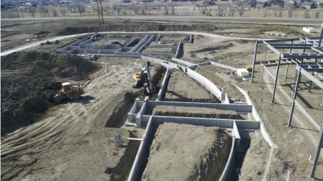
This photo shows the main entrance of the Academic Center and the footings of the Fine Arts Center at the top of the photo.
