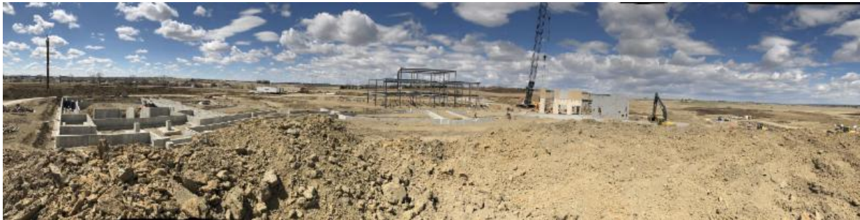
Panoramic Construction View - May 2018
